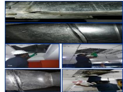
AHU duct leakage rectification by In-house team
